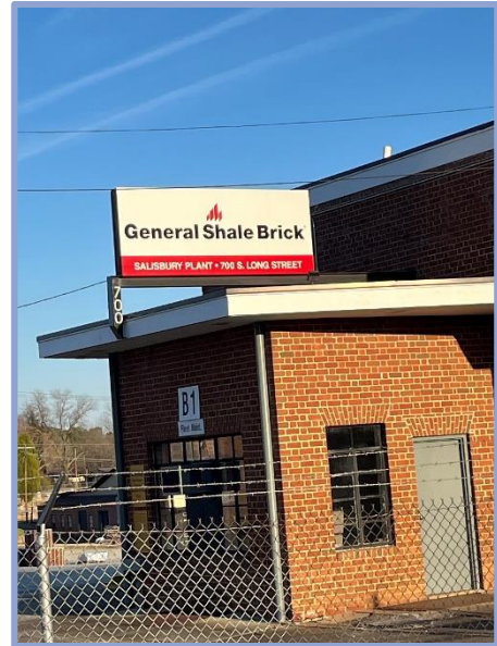
Figure 8: Brick Plant On Long Street
